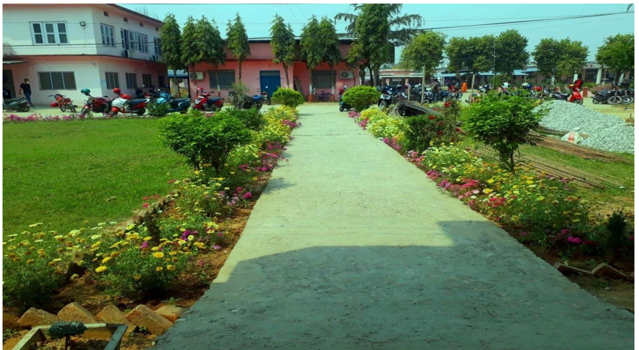
Newly Constructed Er Building
